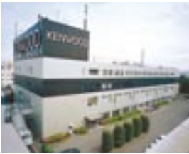
Head Office / Hachioji Business Center
